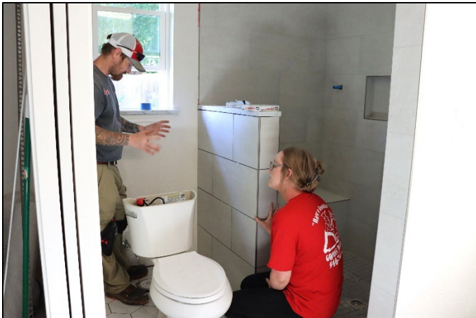
Amanda Latham, WFISD, at Goodin Plumbing
